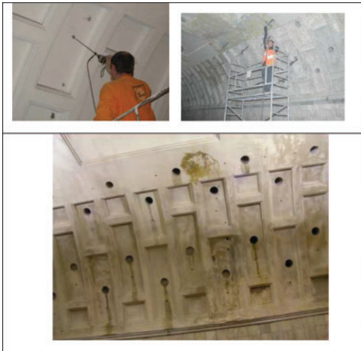
Figure 7. Locating and correcting positions of cementing ports.
